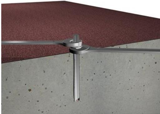
8. Install a stainless steel base plate (BP1), AA407 anchor, M12 washer and clamp down with M12 nylock nut. Tighten the locknut fully and then slack off until the anchor can swivel freely. Ensure minimum of 3 threads are showing.
