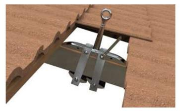
4. Use a hammer to knock the friction plates into compression and tighten the bolts.
