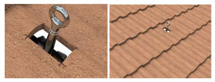
8. Apply Wakaflex or similar flashing over the tile and cut to size with Stanley knife.
