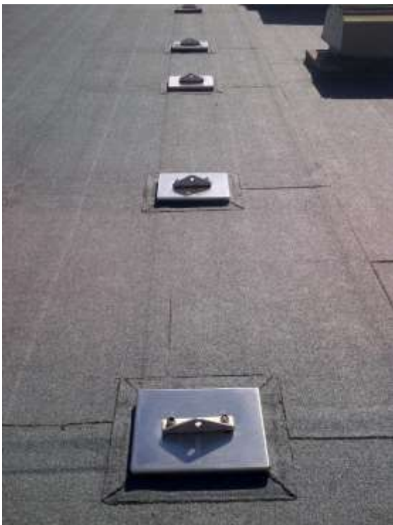
E. Different water proofing technique shown - stainless steel flashing over membrane
