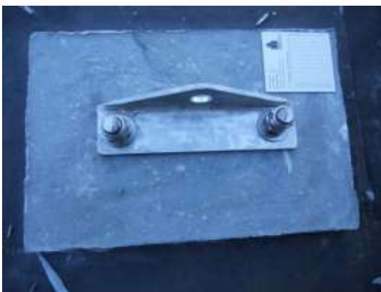
C. Grade 316 stainless steel anchors are installed on the hobs
