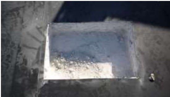
A. Insulation is removed and the slab is exposed
