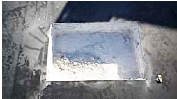
A. Insulation is removed and the slab is exposed
