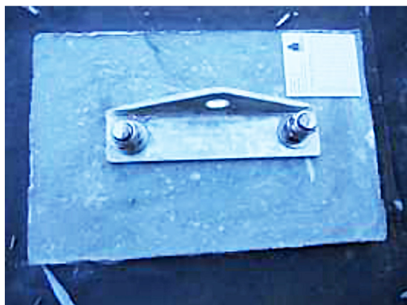
C. Grade 316 stainless steel anchors are installed on the hobs
